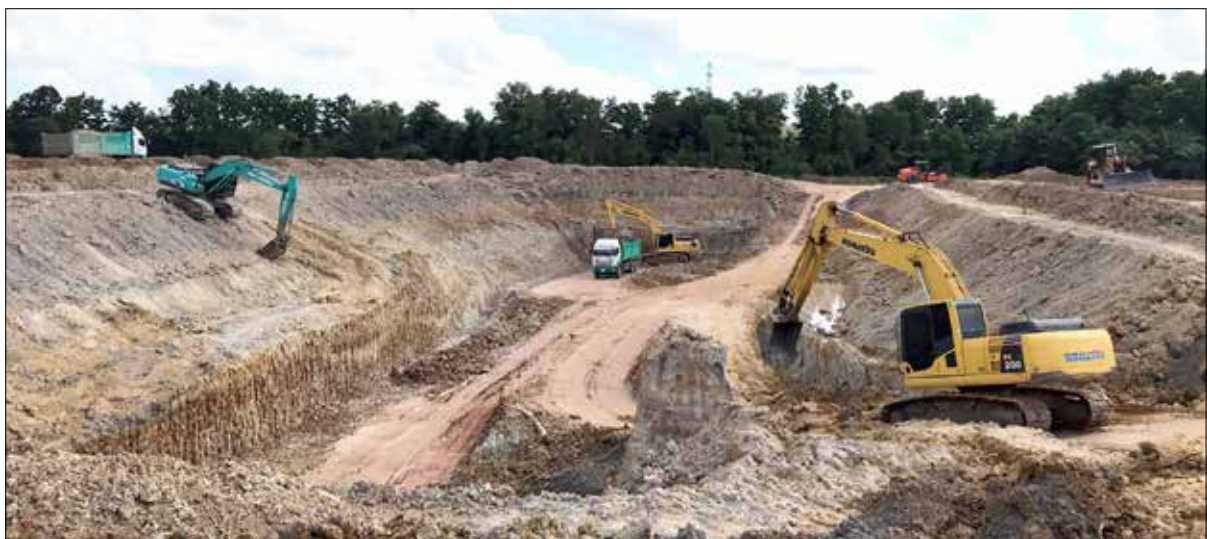
▲ An in-ground biogas digester is now under construction at the Pabon factory. This huge covered in-ground anaerobic creator will hold 40,000 m 3 of Palm Oil Mill Effluent (POME) and will generate methane biogas for renewable electricity.
