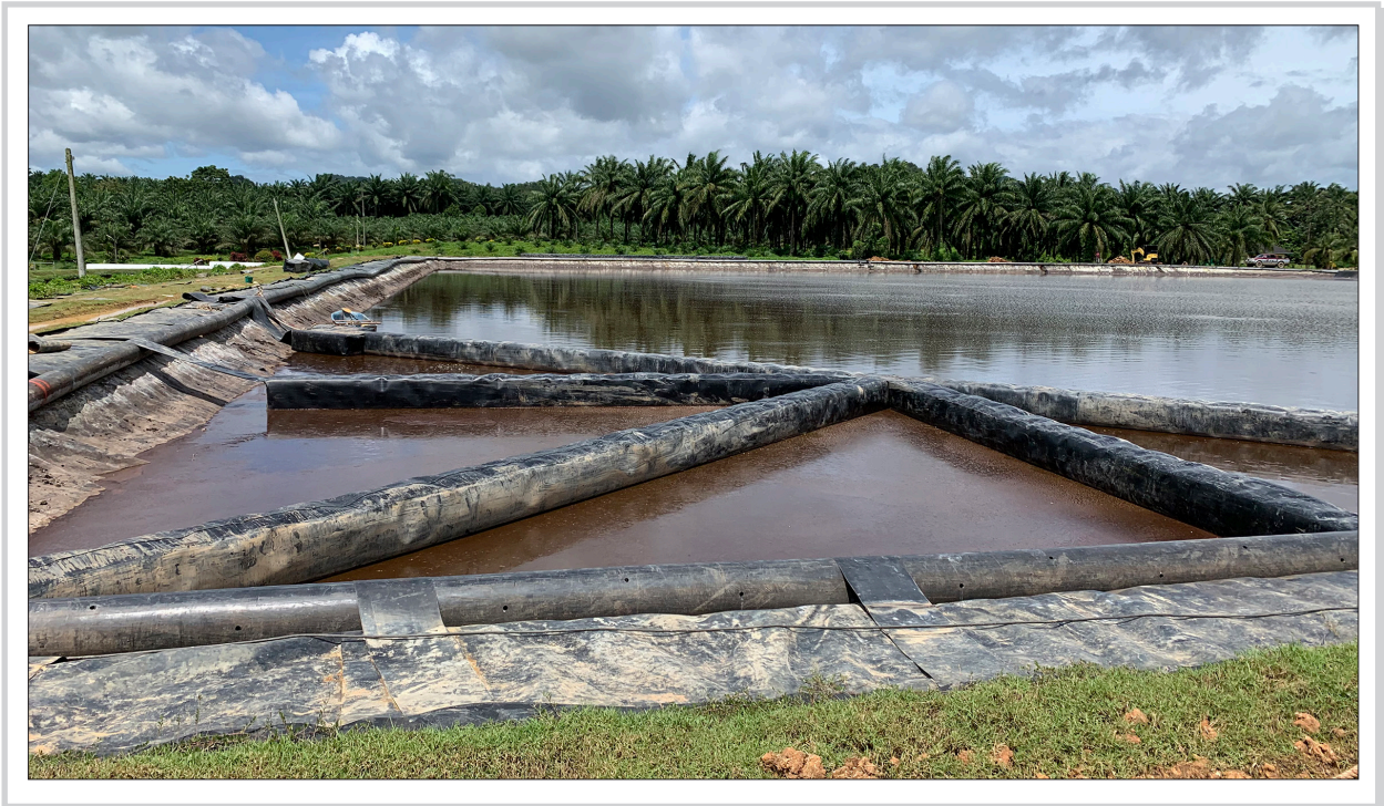
▲ Modifications were made to the in-ground anaerobic reactor.
