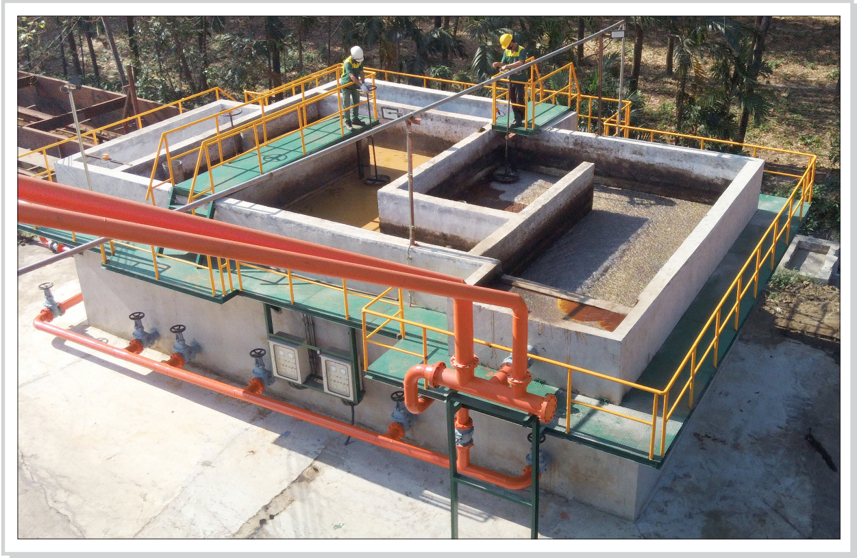
▲ New concrete tank in position with an improved working platform for access and maintenance.
