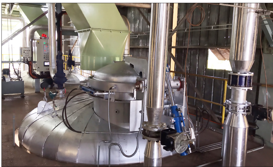
◀ New Steriliser installation.
