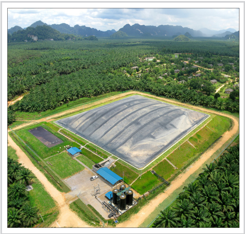
◀ Completion of the replacement cover.
